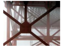
Golden Gate Bridge
